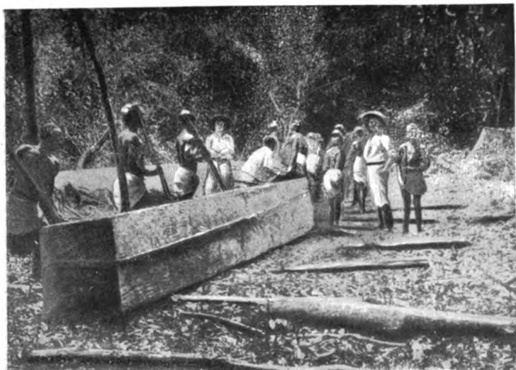
DRAGGING THE SQUARED LOG THROUGH THE BUSH
