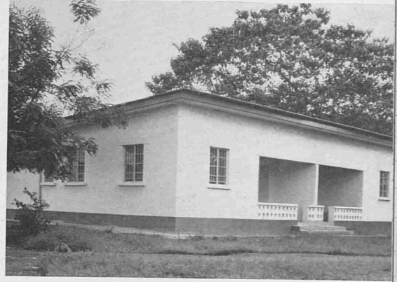
An example of a semi-detached house for African staff of the Sierra Leone Selection Trust
