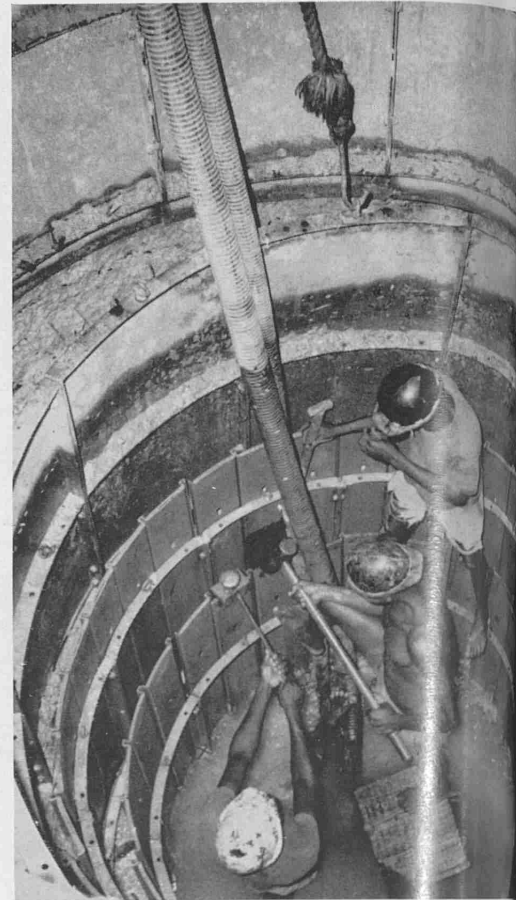
Prospecting for diamonds. A pit lined with metal sections is used for digging through loose soil
